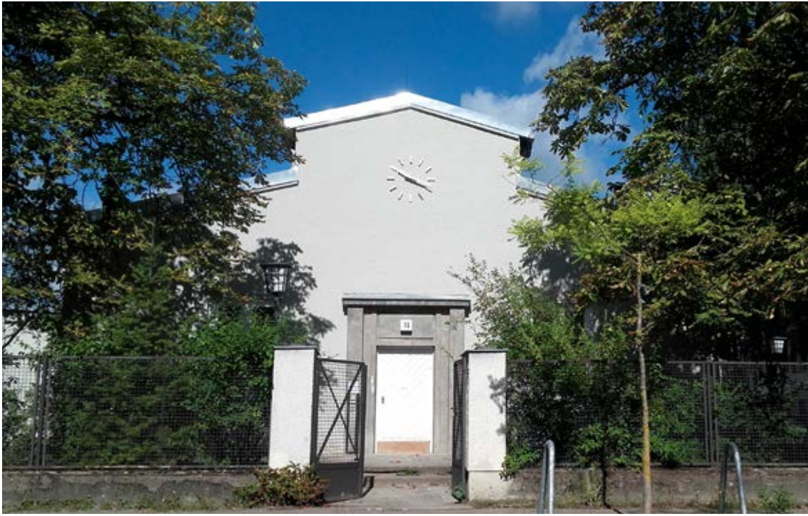
GMPG Research Group, the former "Kältelabor" (Low Temperature Lab) of the KWG, Boltzmann 16 Photo © Schönfeldt
